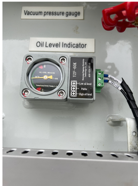
figure 8-16 Oil Level Indicator
