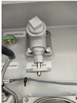
figure 8-20 Oil filling valve
