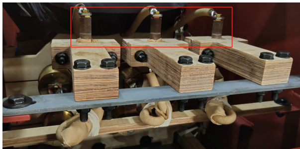
figure 8-11 Replace the fuse
