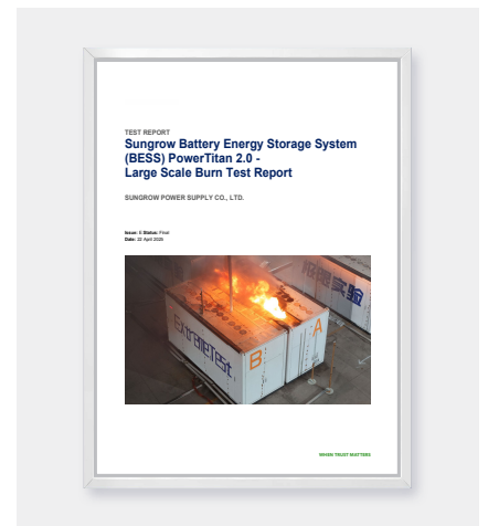
Figure 38: PowerTitan Large-Scale Burn Test Report
