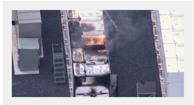
Figure 23: Fire at an Energy Storage Plant in the United States Due to Water Ingress and Short Circuit (Image Source: Mainstream Media Reports)
