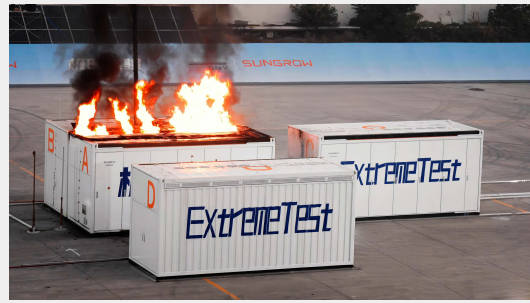
Figure 37: On-Site Large-Scale Burn Test of PowerTitan
