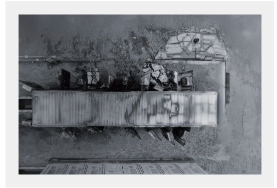
Figure 14: Thermal Runaway Fire Caused by Overcharging Due to 66% SOC Estimation Error at a 20 MWh Energy Storage Station in 2023
