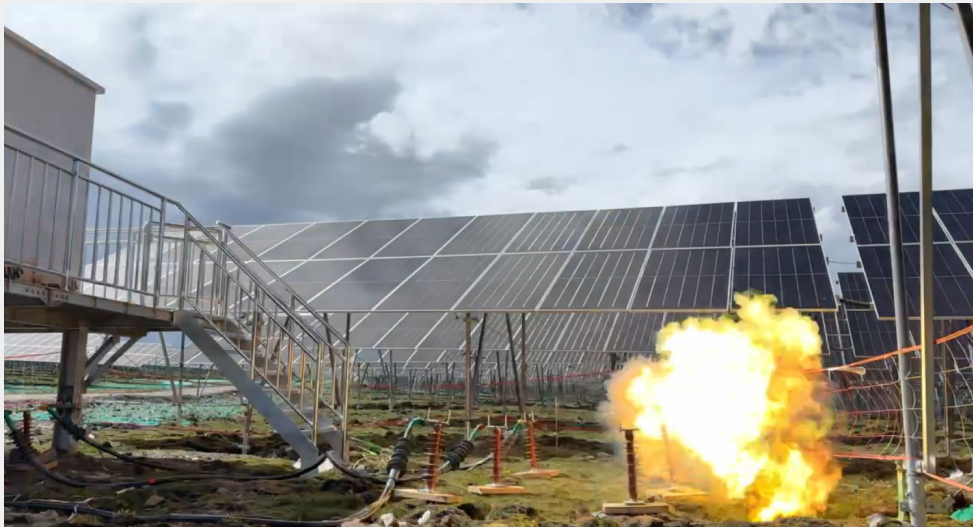
Figure 42: 35 kV Artificial Short-Circuit Test at the Nêdong Caipeng Project in China
